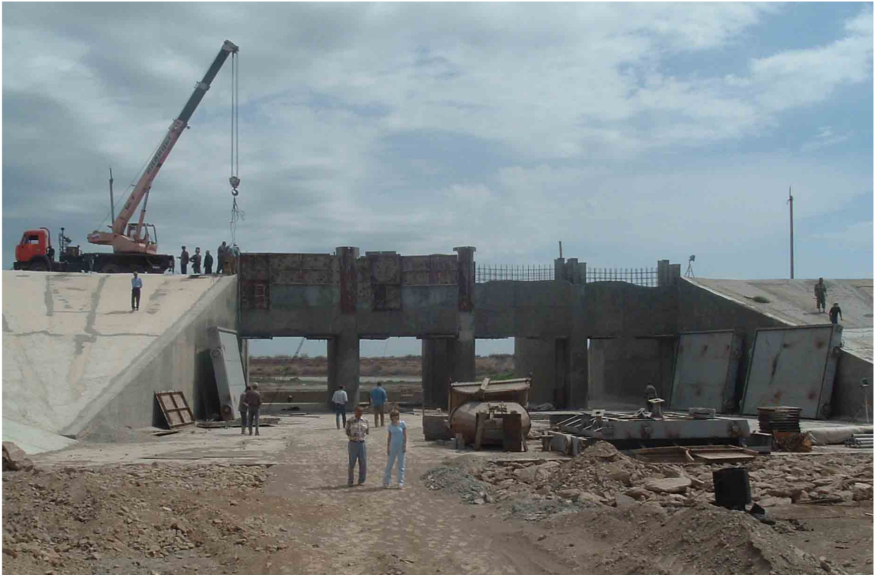
Construction of dam
