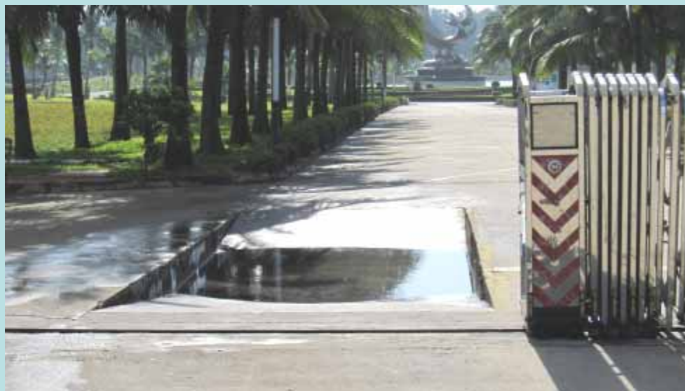
Vehicle washing basin at the gate
